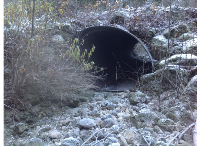
left bank culvert inlet
