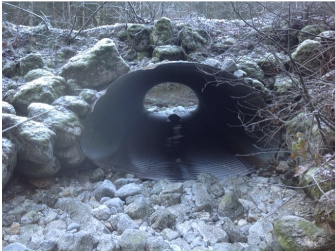
right bank culvert inlet
